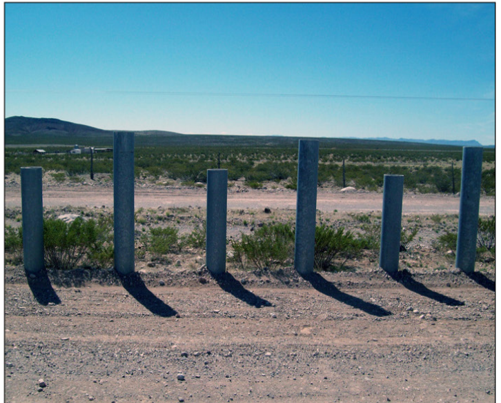
Bollard-style vehicle barrier
